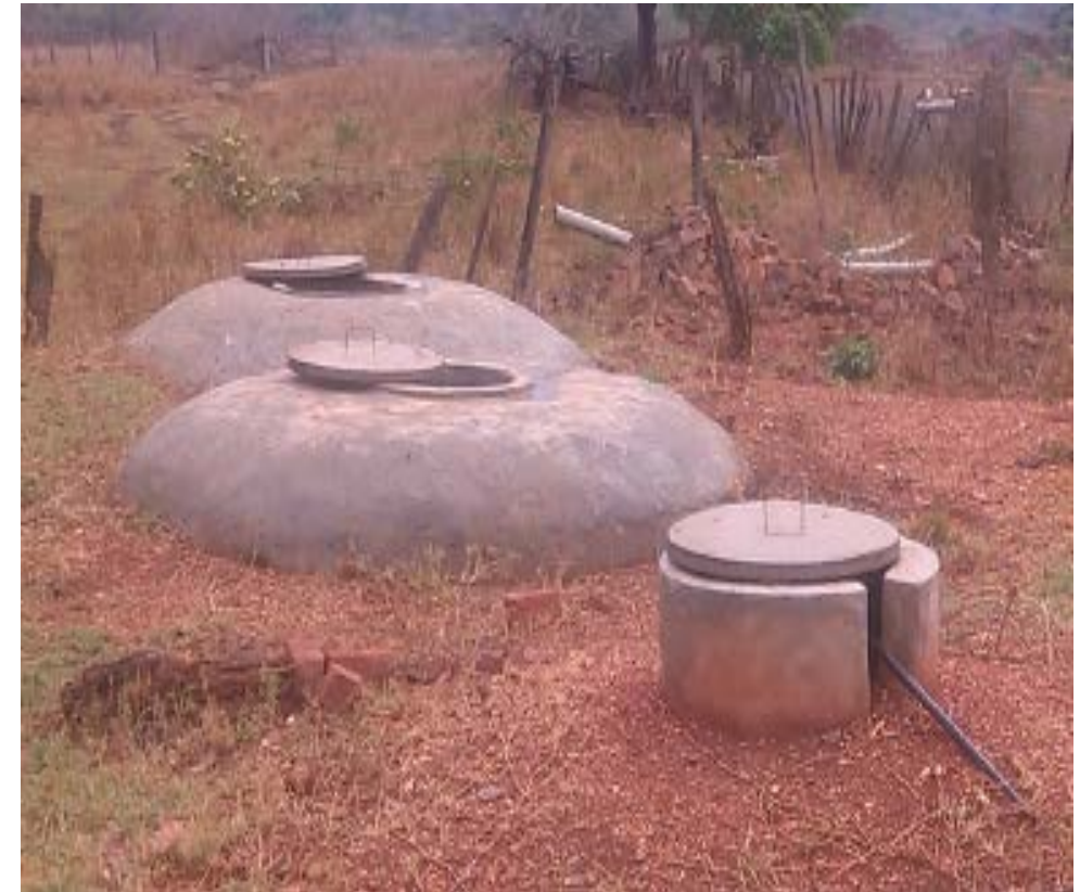
The zero grazed cattle in a Kraal and a fixed dome biogas digester
