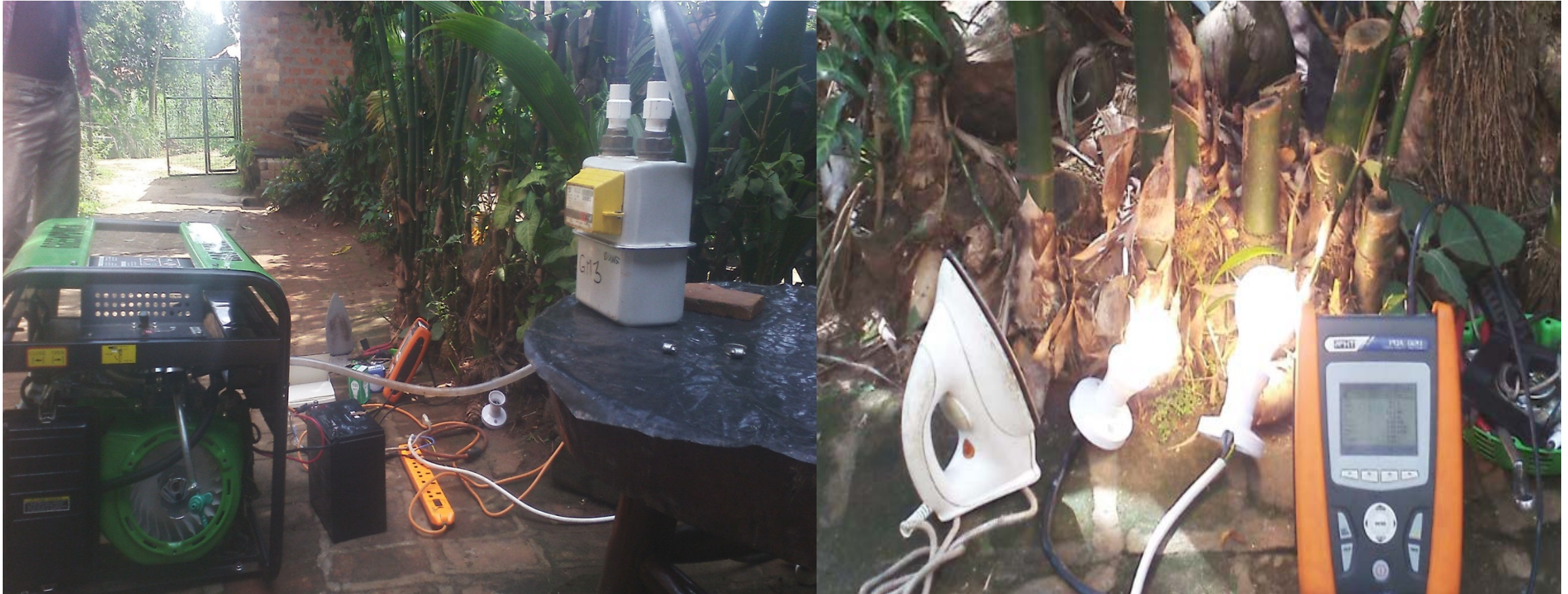
The 3kW gas-engine with a gas meter and the electric loads under test
