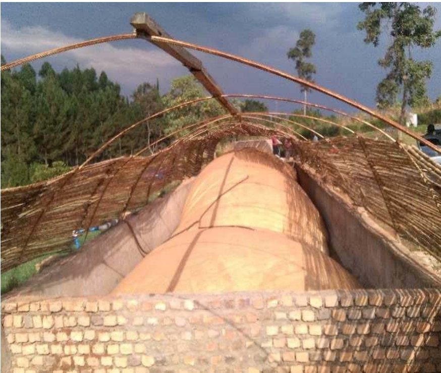
The plug flow (PVC material) digester and a gas-engine generator
